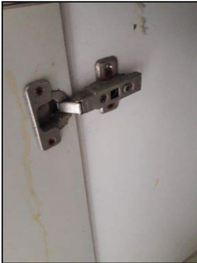
Rusted cabinet panel hinges
