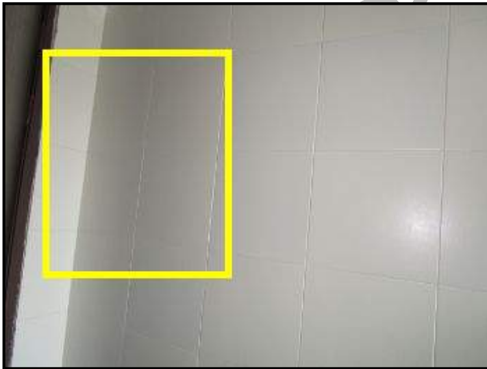
Tiles of different shades installed
