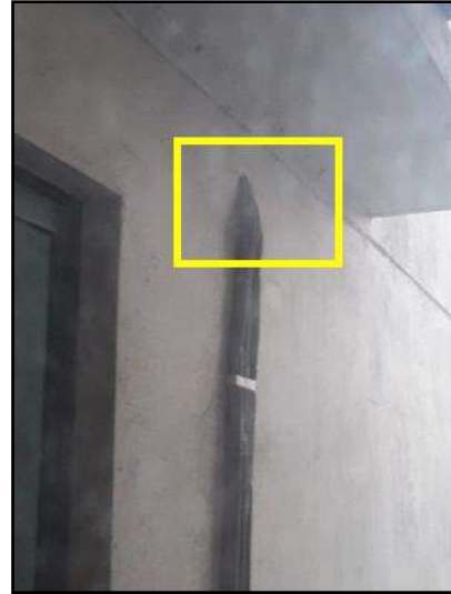
Packing note done around AC pipe sleeve
