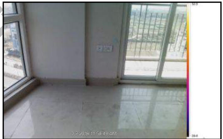
Visual Image of Bedroom 1 front wall
