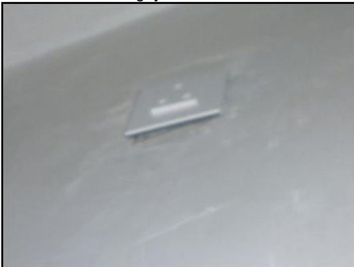
Geyser socket point concealed casing is up mounted at one side
