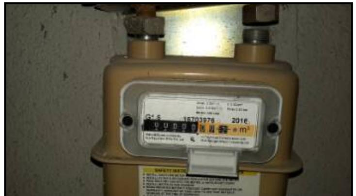
Lpg meter has not been installed properly
