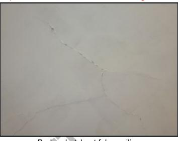
Broken hatch at false ceiling
