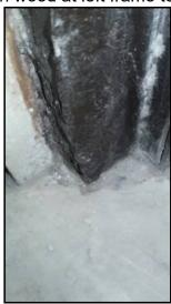
Improper finish at right frame bottom side
