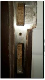
Screw missing at groove
