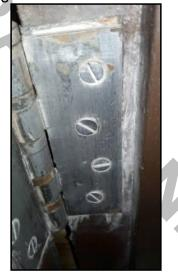
Right frame bottom hinge has not been installed properly
