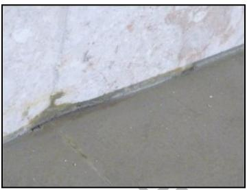
Gap between wall tiles and floor tiles at left wall wet floor
