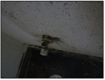
Water tap valve improperly installed at right wall
