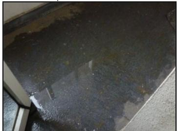
Water accumulation observed at middle of floor due to improper slope
