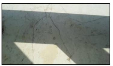
Multiple cracks at marbles at railing sill top at balcony
