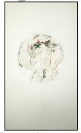
Improper finish at left wall around electrical circular point
