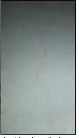
Vertical crack at back wall above door frame
