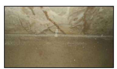
Crack at back wall bottom side behind door
