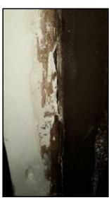
Improper filling at frame and wall inside
