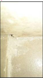
Gap at floor and wall at back wall
