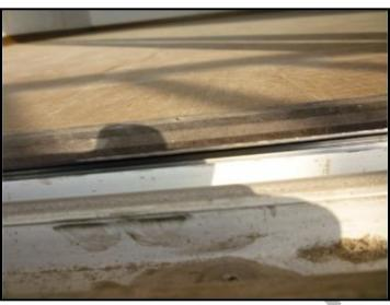
Floor transition improperly installed at sliding door as having gap with sliding door's bottom channel
