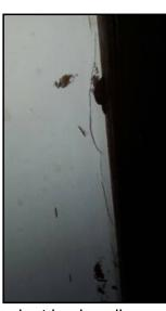
Vertical crack at back wall near left side of bathroom door frame
