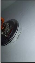
Improper finish around sprinkler at right wall
