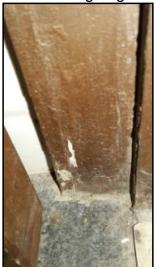
Crack at right frame bottom side
