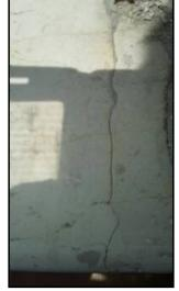
Multiple cracks at marbles at railing sill top at balcony
