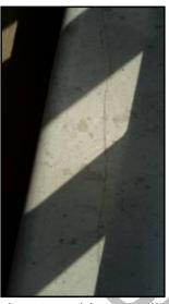
Multiple cracks at marbles at railing sill top at balcony
