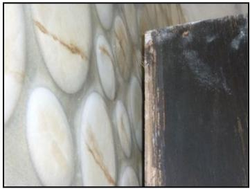
Gap between wall and cabinet at top left corner due to improper installation
