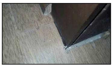
Gap at floor laminate and bathroom 1 door frame
