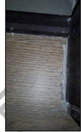
Gap at floor laminate and bathroom 1 door frame
