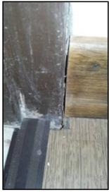
Gap at beading and frame and at flooring and frame
