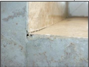
Improper filling at left window sill corner
