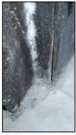
Gap at right frame joints at bottom side
