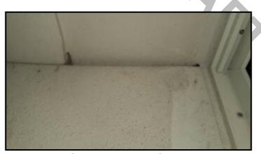
Gap at duct and left wall
