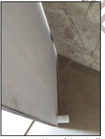
Improper position of door buffer
