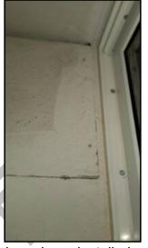
No screws have been installed around duct
